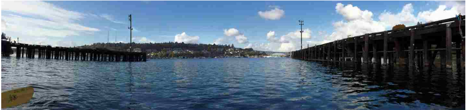
Figure 20. View looking west, between the two piers.
